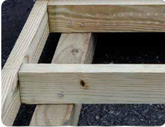
Pressure Treated 2x4 Floor Joists 4x6 Runners
