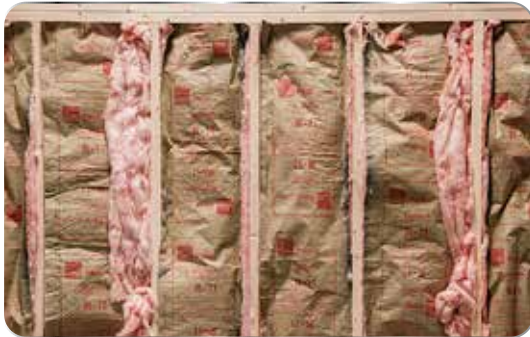
R-13 Batten Insulation In Walls & Ceiling
